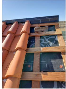
to check the underlayment while doing these repairs, because if the underlayment is deteriorated or will need replacement soon, then it may be advisable to replace the furring strips and underlayment at one single time in order to save on costs in the future.
