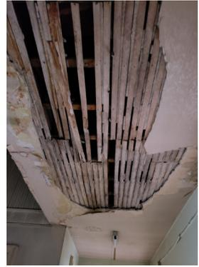
Sometimes where there are enough intermittent repaired cracks and/or missing sections of plaster, it will warrant a new plaster “skim coat” over the entire wall surface to give it a uniform texture.
