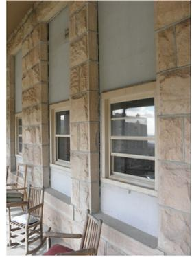
which can give the appearance of glass on the exterior and a wall can be installed on the interior to block the window from the interior side, but note to properly insulate the cavity between the window and the wall in this scenario.
