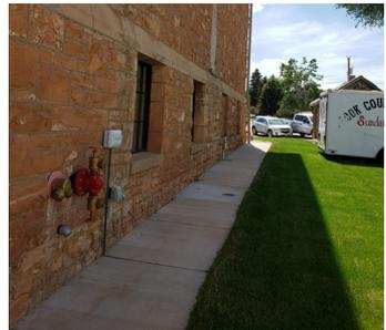
Some jurisdictions and some circumstances (some residential uses) may allow a single water line to serve both the domestic water system, as well as, the fire protection system. However, many jurisdictions and circumstances require a separate fire protection water line from the domestic water line, requiring a separate water tap within the street.
